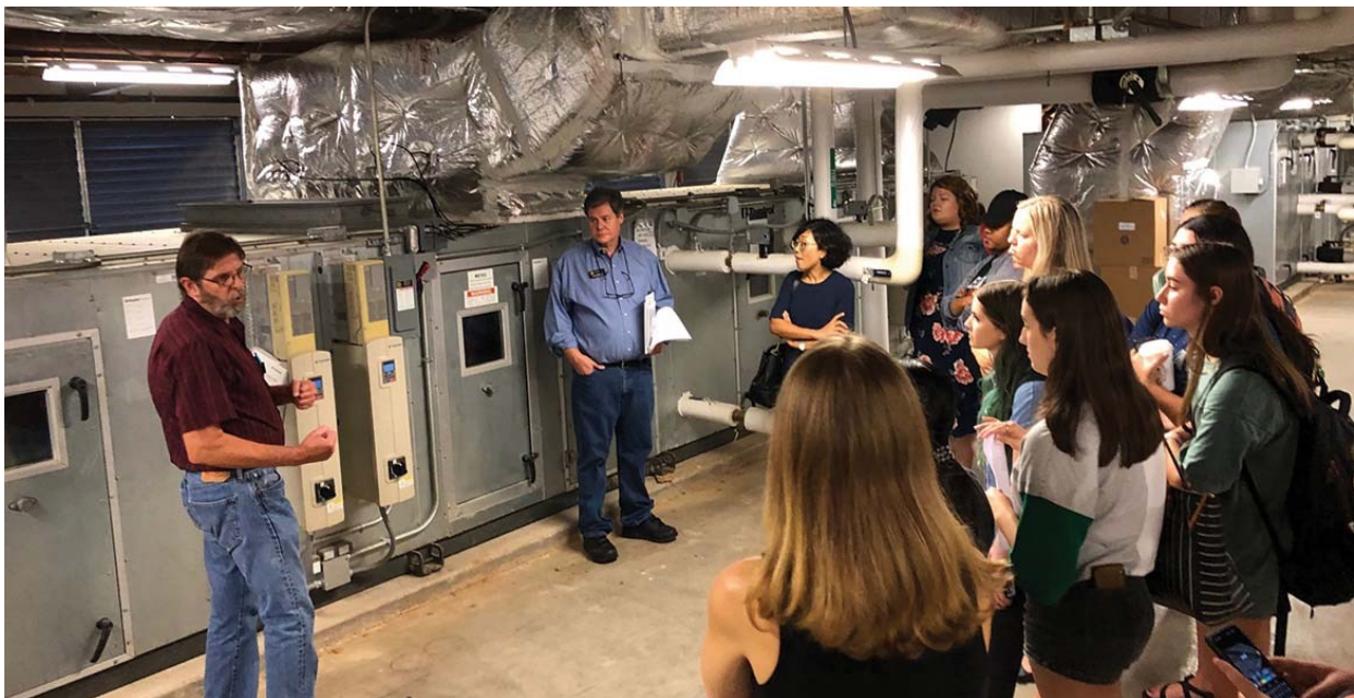
Steve Ledbetter, left, gives a behind-the-scenes tour of a mechanical room in Human Sciences, Facilities Management Zone 2.
